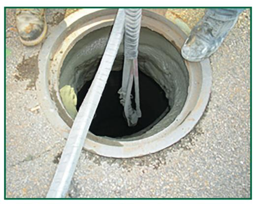
A variety of cementitious products were evaluated and Permacast MS 10,000 made by AP/M Permaform was selected for all manhole and catch basin relining.
