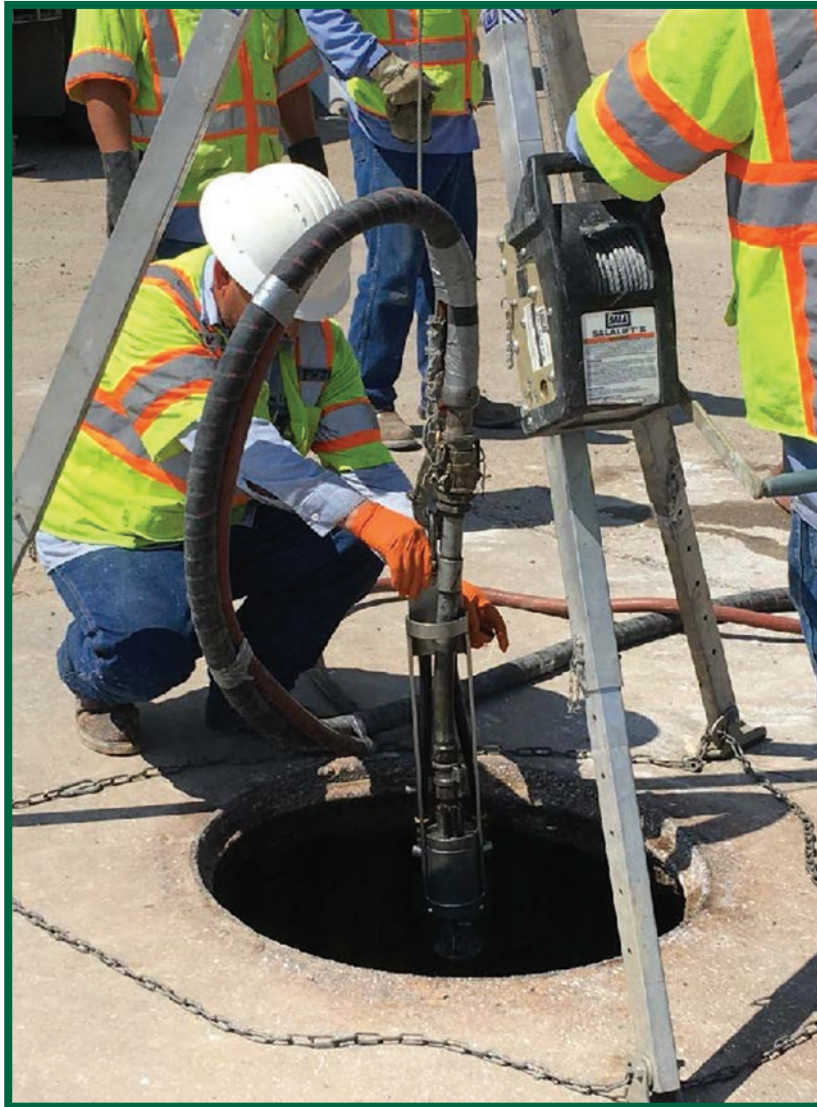
City of Laredo crew rehabilitates with one-step above ground process
