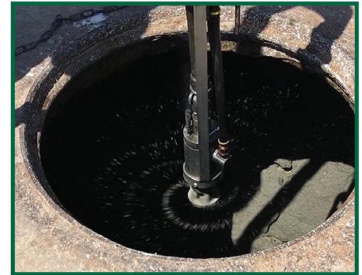
Manhole spincasting with Permacast system
