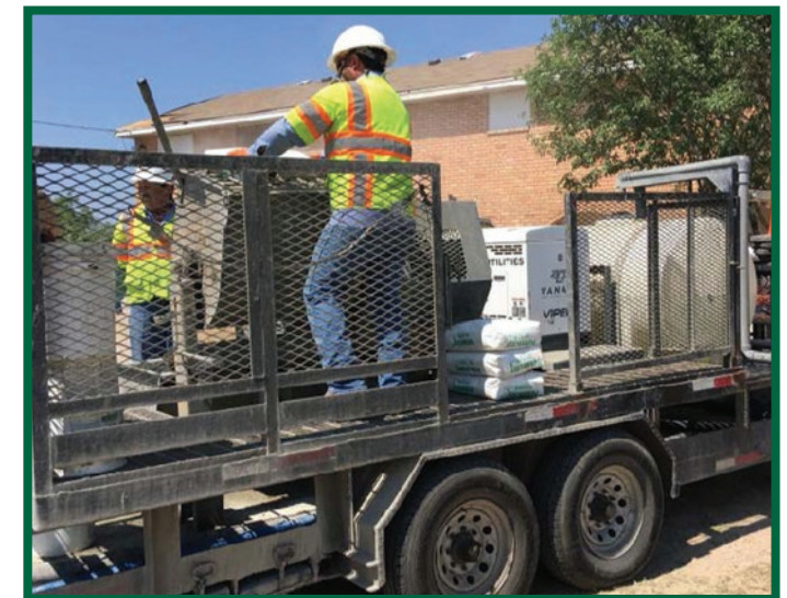
City of Laredo manhole renewal trailer
