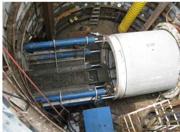
Figure 6: Pipe ramming 96" ConShield-protected concrete sewer tunnel in MSD
