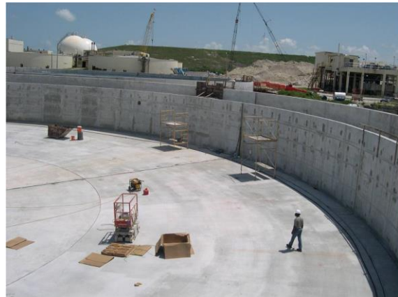
Figure 5: Completed section of upgraded Black Point facility
