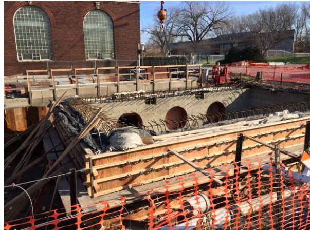
Figure 8: Construction of the new combined-system culvert begins
