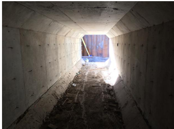
Figure 10: Completed Con mic Shield-protected HSD box culvert
