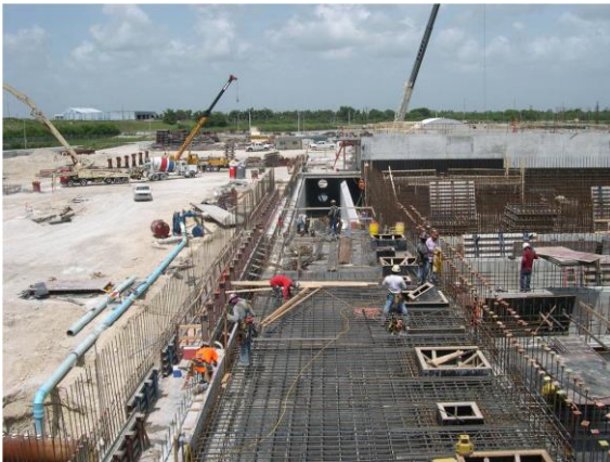
Figure 4: Construction of Black Point Wastewater Treatment Plant upgrade and expansion
