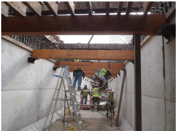
Figure 9: Preparing to pour the top of the pipe in place
