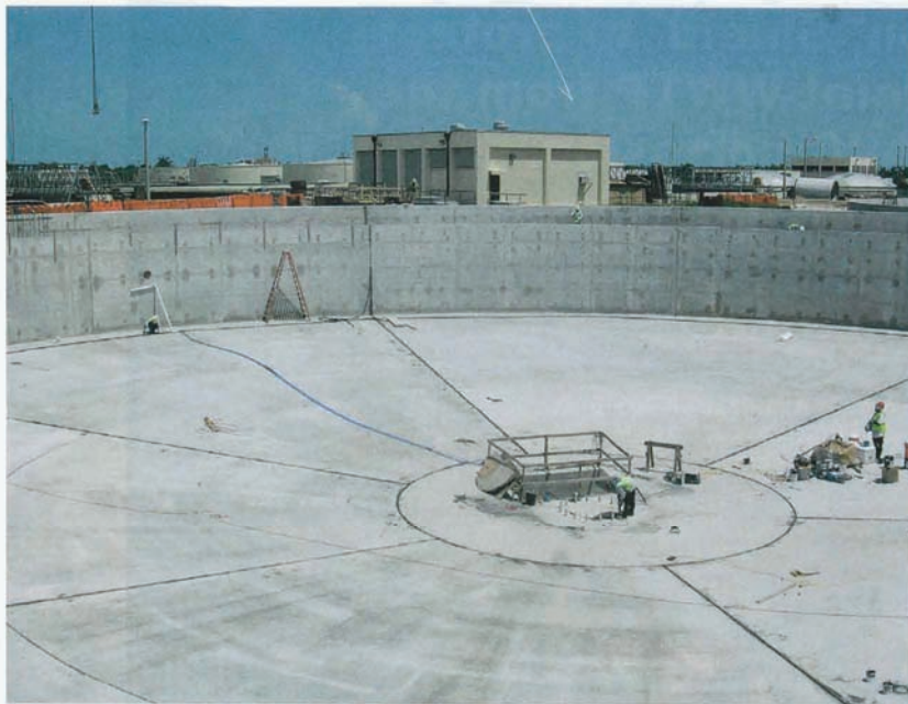
The ConShield antibacterial additive is mixed with concrete at the batch plant. A clarifier at the Black Point plant is shown under construction using the treated material.
