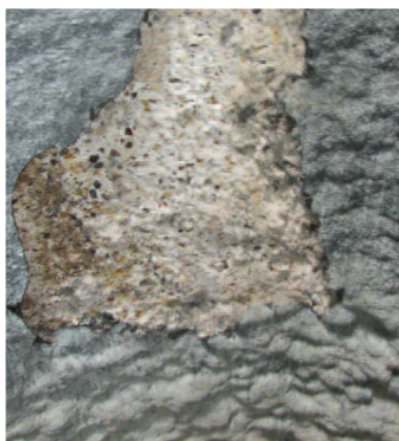
MIC delamination of coated manhole
