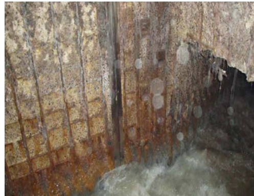
Figure 4 Reinforcing steel exposed after pressure washing
