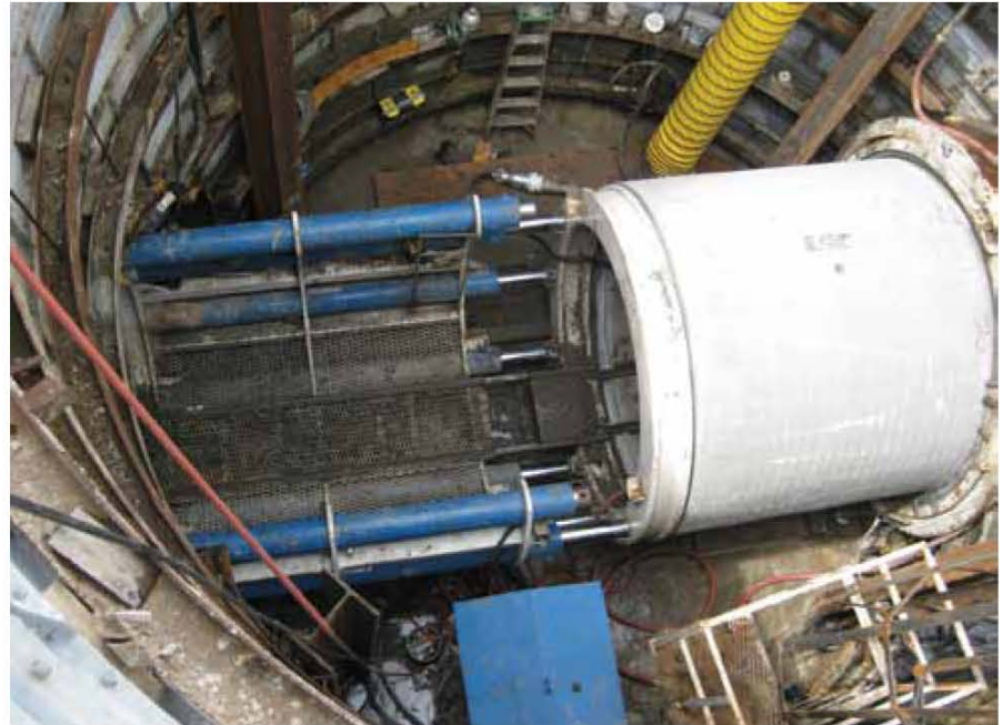
Concrete was selected because of its ability to withstand the jacking forces and depth of bury for this project.
