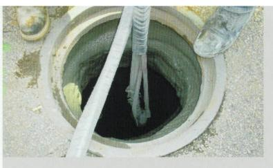
enhanced MS 10,000. The epoxy-coated, cement-reinforced manholes represent the state-of-the-art in manhole rehabilitation and are expected to last another 100 years.
